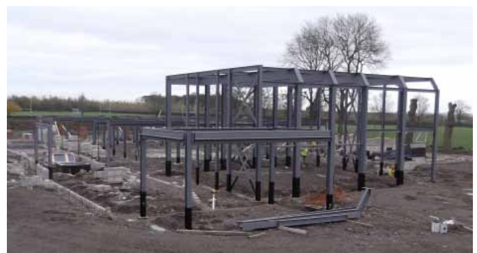
The construction work begins in earnest
